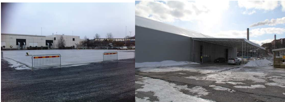
Figure 9: Construction of BLC, winter 2012/2013
