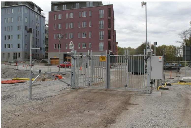
Figure 8: The photo above shows a folding gate with a radio LAN mast and camera surveillance
