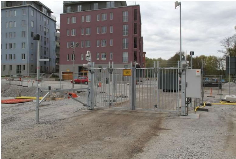
Figure 8: A folding gate with a radio LAN mast and camera surveillance
